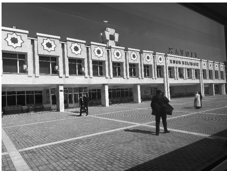
Navoiy Train Station
