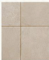
Even grout lines
