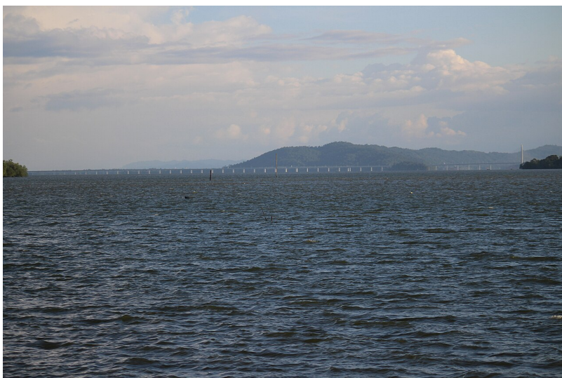
Figure 25: The Sultan Haji Omar Ali Saifuddien Bridge, which crosses Brunei Bay to connect the Temburong enclave with the rest of the country. Opened in 2020, it is one of Southeast Asia's longest bridges. Source: Wikimedia Commons, CC BY-SA. URL: https://commons.wikimedia.org/wiki/File:Sultan_Haji_Omar_Ali_Saifuddien_Bridge_08.jpg
