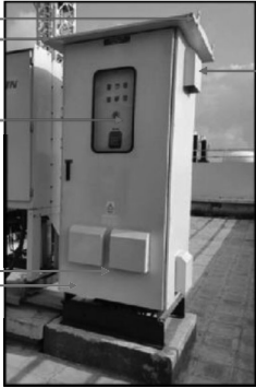
IP 54-VFD PANEL GENERAL ARRANGEMENT
