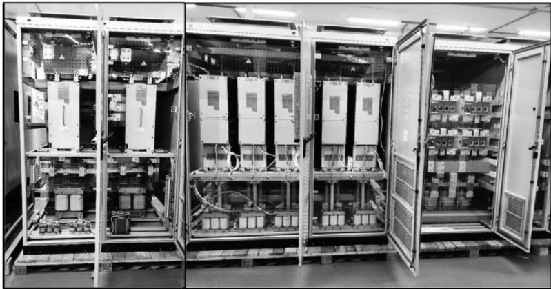
IP 42-5 AXIS MULTI VFD PANEL GENERAL ARRANGEMENT
