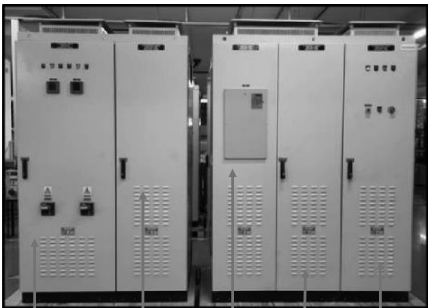
Incomer converter Control Cubicle Cubicle module Inverter Control & motor Cubicle termination
