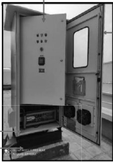
IP 54-VFD PANEL GENERAL ARRANGEMENT
