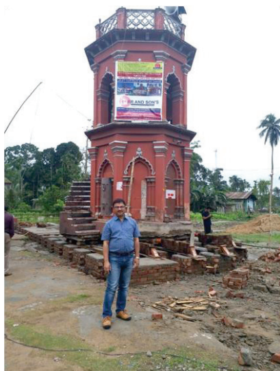
Shifting of Minaret of Puranigudam Masjid due to extension of the National Highway
